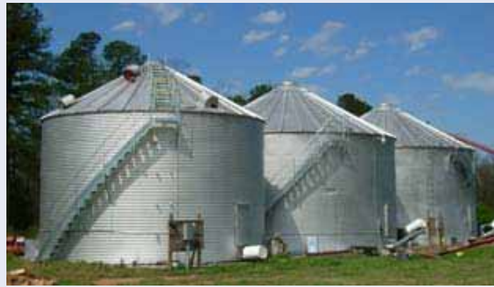
Grain bins showing stairway installation in progress
