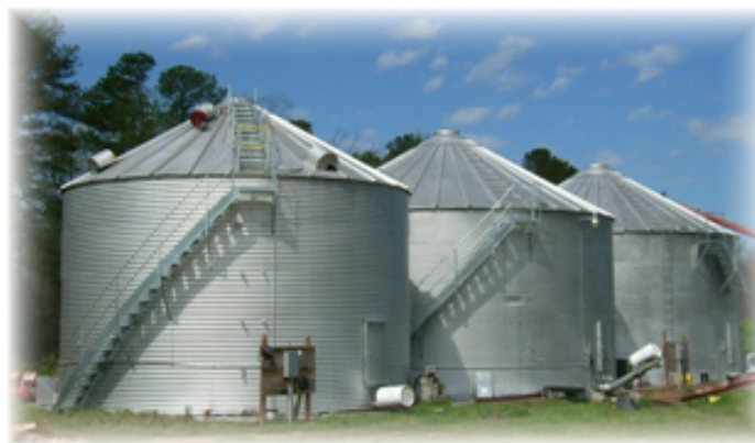
Grain bins showing spiral stairway installation in progress
